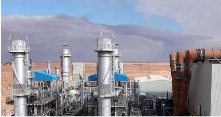
Figure 5. Hassi R'Mel power plant.
