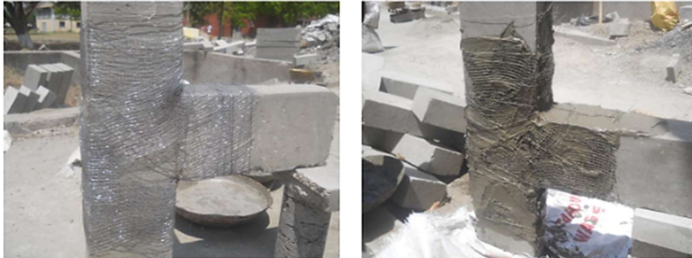
Figure 1. Application of Ferrocement Jacket
